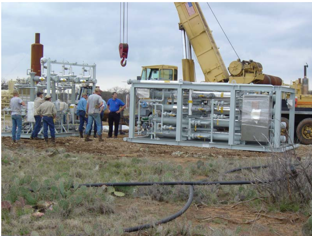
Figure 3. Membrane system being installed at Green Ranch, TX.
