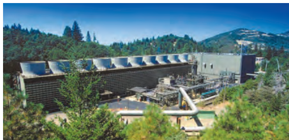
One of Calpine's 15 geothermal power plants at The Geysers, the Big Geyser plant has an installed capacity of 97 megawatts. Big Geyser has been in operation since 1980 and is a dry steam-type geothermal power plant. Photo from Calpine Corporation, NREL 17270
