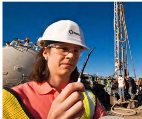
An NREL senior geothermal analyst examines a heat sensor order before the wire attached to the sensor descends 500 feet under the new IKEA store construction site in Centennial, Colorado. The new store relies on geothermal heat pumps to supply much of its heating, cooling, and hot water needs. Photo by Pat Corkery, NREL 17907
