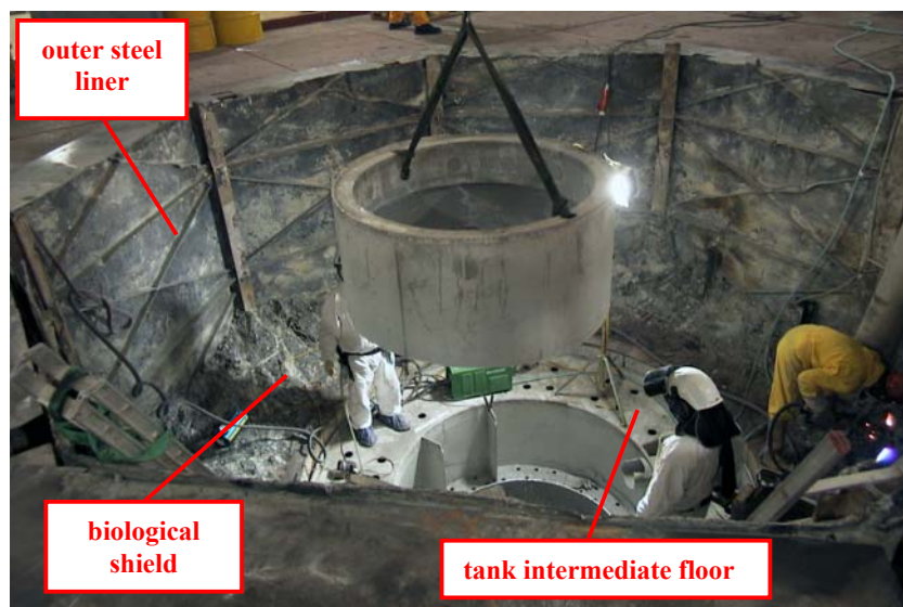
Fig. 3 Dismantling the upper section of the reactor block
