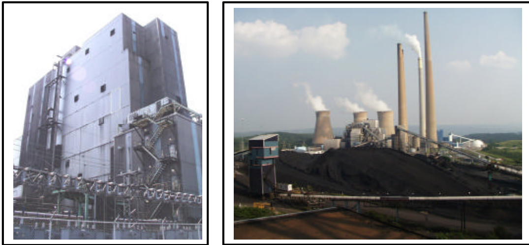
Edison Mission Energy's 1,100-tph Homer City Coal Processing Plant (left) provides clean coal to its adjacent 1,850-MW Homer City Power Plant.
