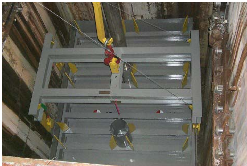
Fig. 4. Sludge Storage System in T Plant Cell
