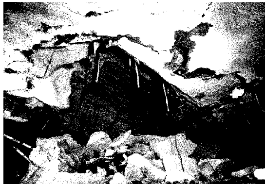
Fig.1 The blocky nature of the rock mass is evident in the collapse of this cavern in Tuff.
