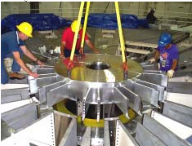
Figure 6 Transition high-voltage conductor installation
