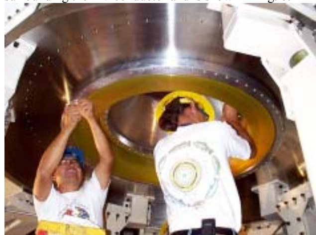
Figure 8 Bottom insulator installation
