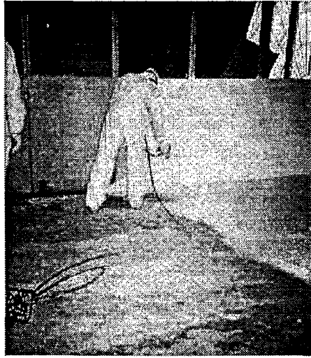
Figure 2. Russian technical expert spraying the concrete floor of the loading dock in the high-bay area.
