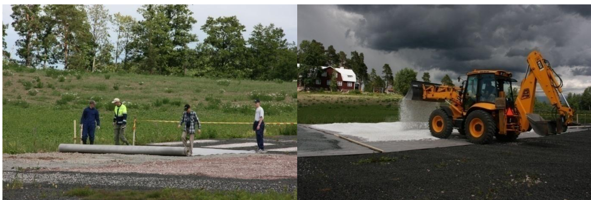
Figure 3. Construction of a test field of gravel. The root blocking carpet is installed (left) and a 5–10 cm layer of gravel spread over it (right).
