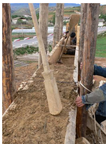
Figure 11. New rammed earth building in Shangri-La (Zhongdian) County, Yunnan. Rammer detail [17].
