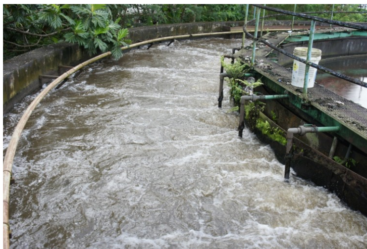
Figure 5. Contact-stabilization type activated-sludge wastewater treatment plant on Pohnpei. Image source: author.
