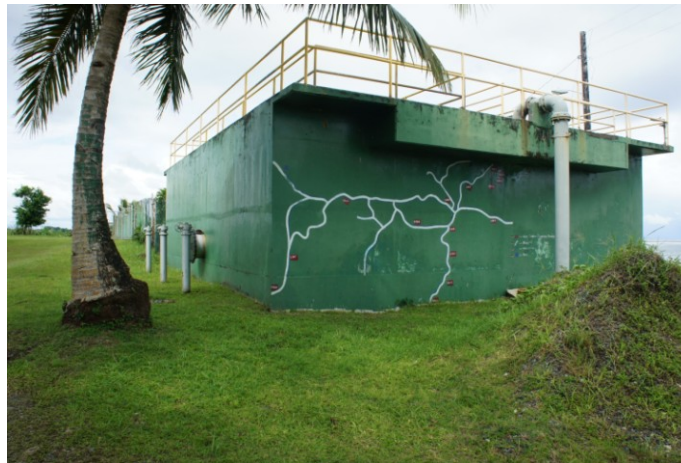
Figure 8. Imhoff tank wastewater treatment plant in Colonia Village, Yap, with a map of the sewer network painted on wall. Image source: author.
