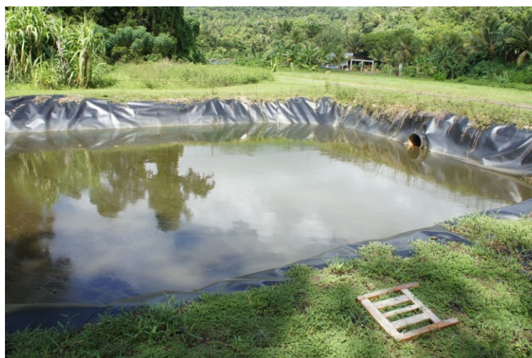
Figure 4. Lined leachate catch pond at the “Fukuoka-type” landfill on Kosrae. Image source: author.
