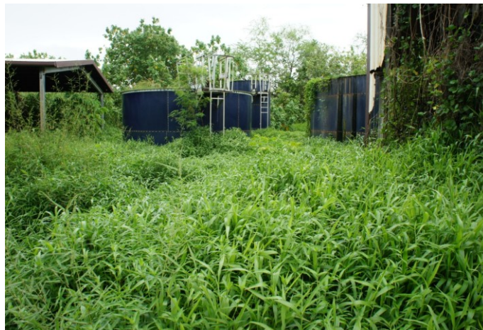
Figure 6. Inoperative industrial wastewater treatment plant of tuna-packaging plant on Pohnpei. Image source: author.
