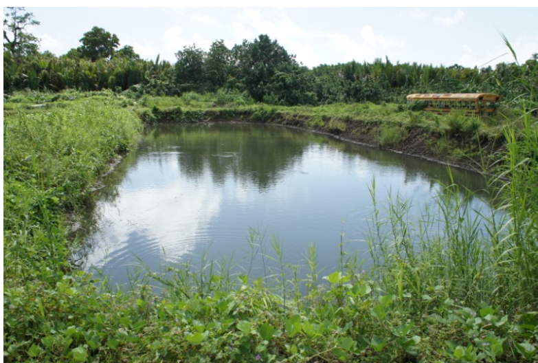
Figure 2. Wastewater treatment system in Kosrae consisting of three oxidation ponds (only one pond shown). Image source: author.
