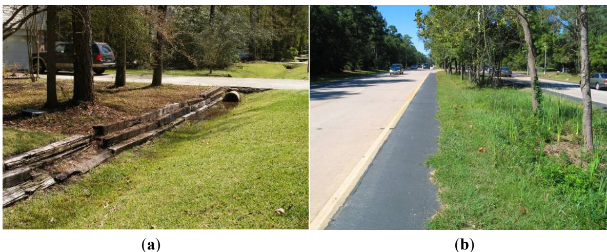
Figure 2. (a) A typical view in The Woodlands: preserving the original vegetation, minimizing turfgrass areas, and using open surface drainage; (b) A typical collector street in The Woodlands: stormwater drains to the vegetated medium for treatment.
