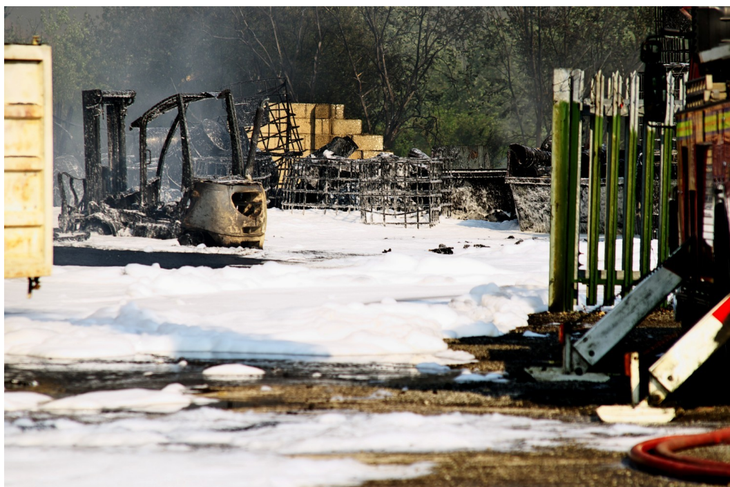
Figure 2. Example of an industrial estate polluted by foam-based firewater runoff during the day (photograph provided by Ian Duckworth).
