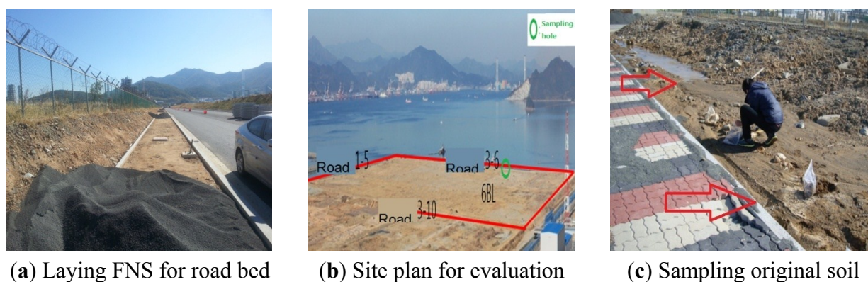
Figure 3. Construction of FNS and sampling of the original soil at the sidewalk at the Yeosu Oil and Chemical Pier.
