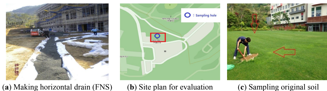
Figure 4. Construction of the FNS and sampling of the original soil at the front plaza of the Suncheon Lakehills Golf Club.
