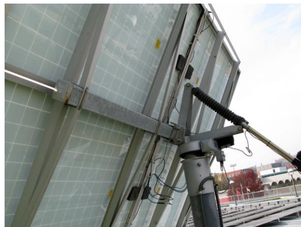
Figure 6. Examples of solar panels that follow the sun, on NJIT's roof. In this example, also, the energy flow from solar to consumption can be process modeled relatively easily.
