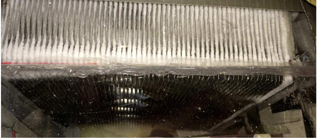
Figure 6: Heat exchanger 2 at time of minimum resistance with frost starting to build up between fins at the top
