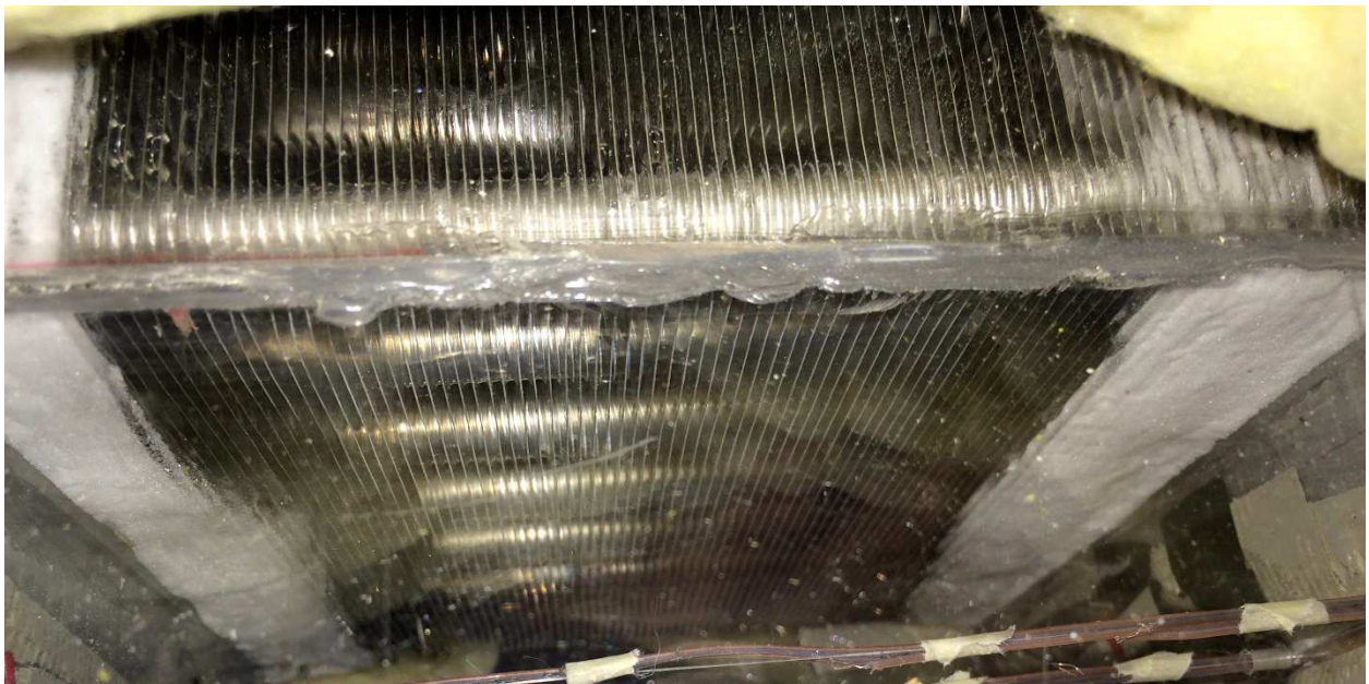
Figure 7: Heat exchanger 3 with excessive frost buildup from the sides
