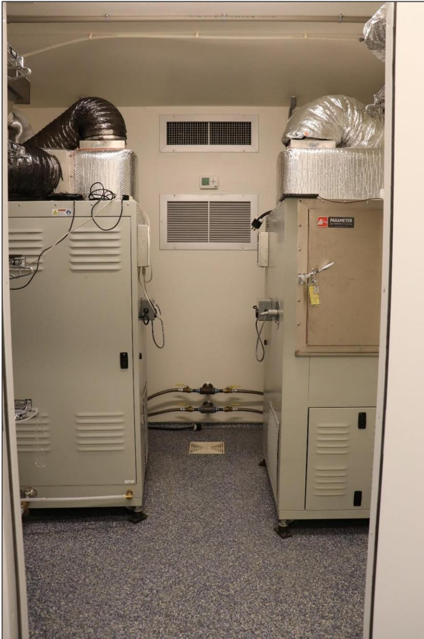
**Figure 3.9.** Parameter Generation and Control (PGC) unit inside the equipment rooms.
