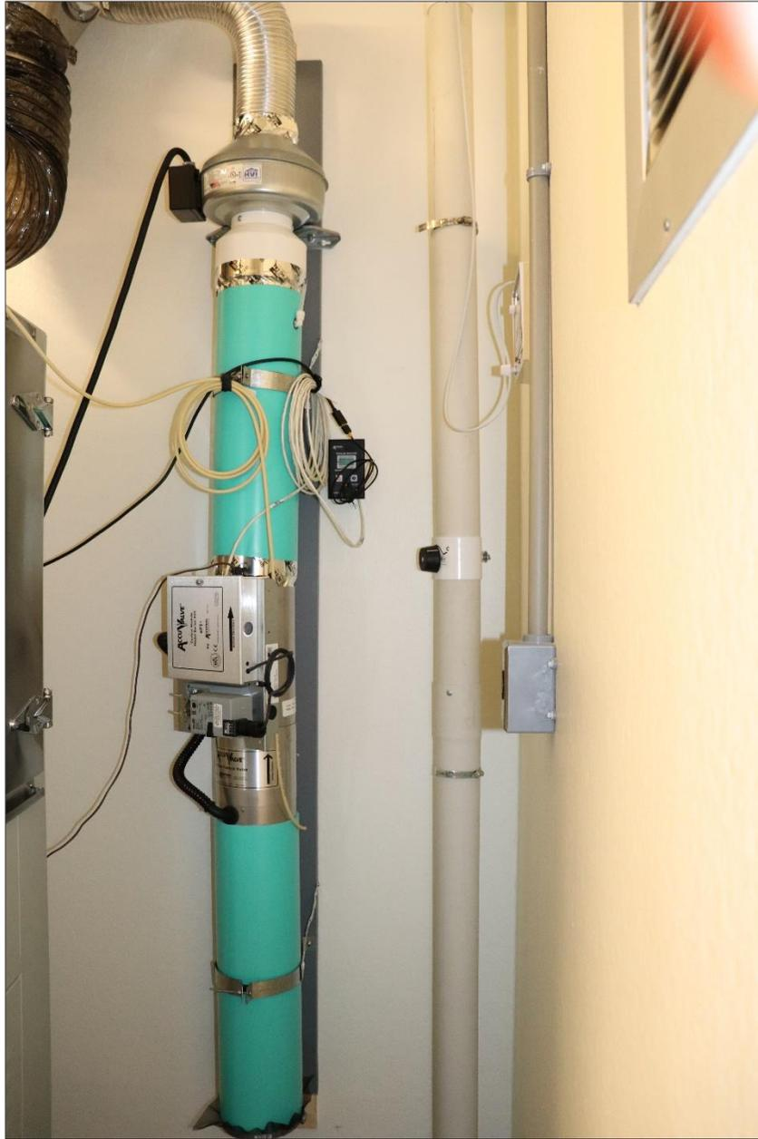
**Figure 3.11.** Fresh air supply system.
