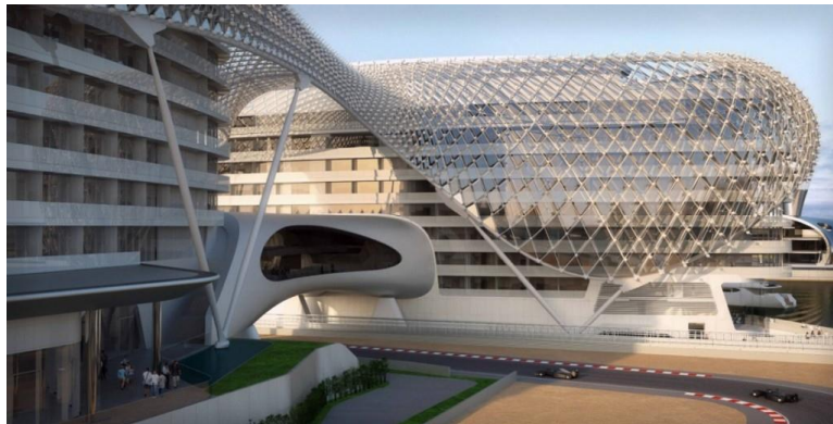
Figure 3. Example of projects of reticulated shells of arbitrary configurations
