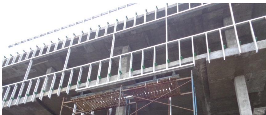
Figure 1. Cold-formed steel walls at the construction stage.
