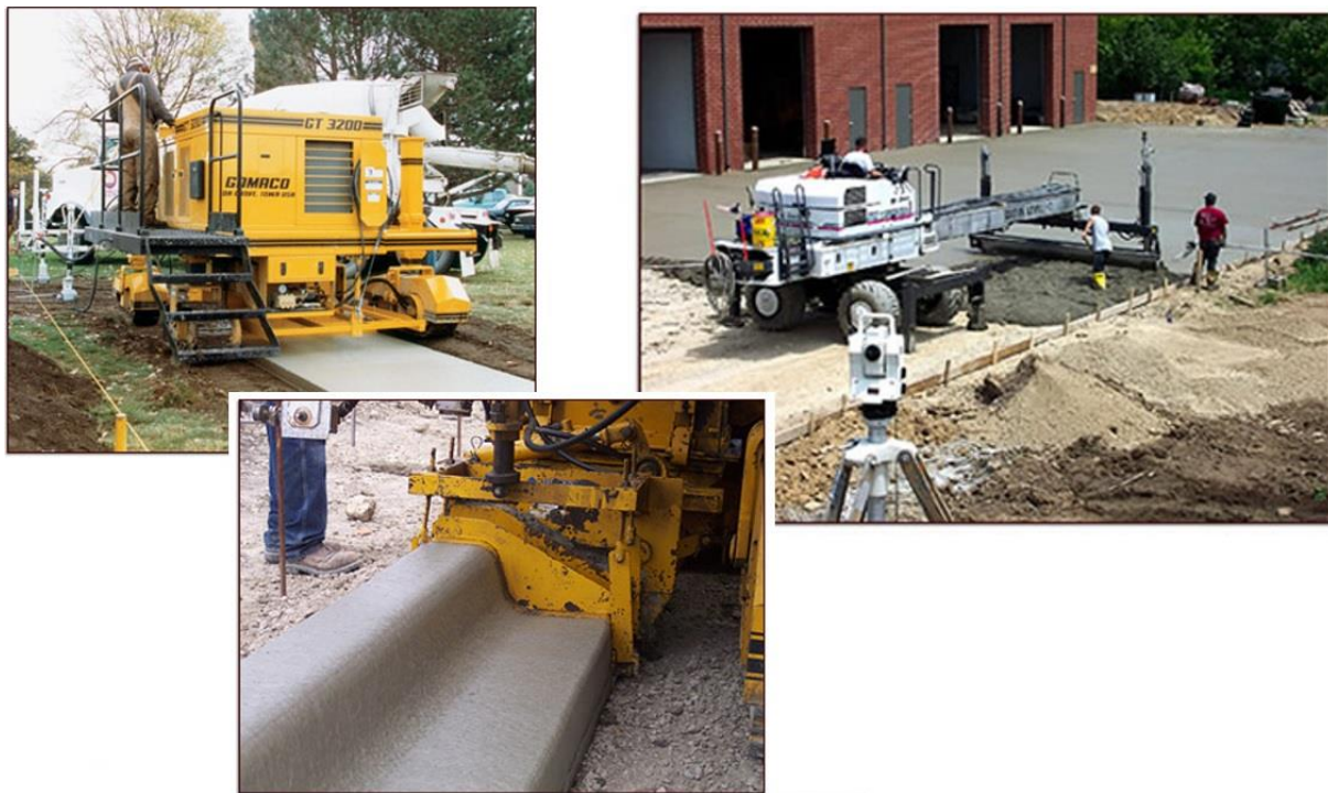
Figure 3. Laser 3D technology of concrete pouring.
