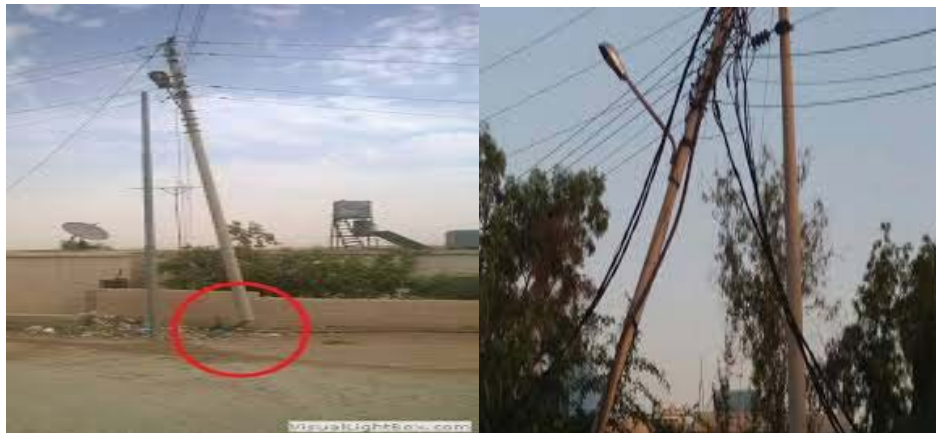
Figure 1. Corrosion effected on the lower part of the electrical poles
