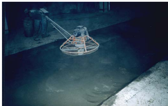
Figure 2. Technology of monolithic magnesium flooring.
