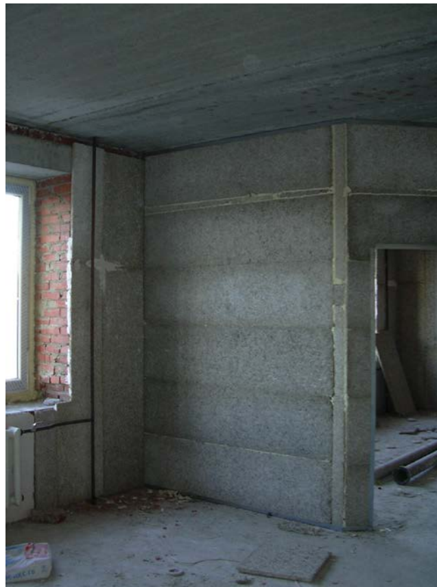
Figure 1. Application of materials based on magnesium oxychloride cement as a heater.
