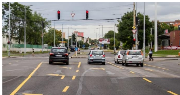
Fig. 5. Use glued traffic markings on the road but can see the old ones
