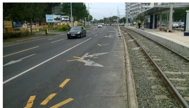
Fig. 3. Traffic lanes and road markings are "slip" from the original place
