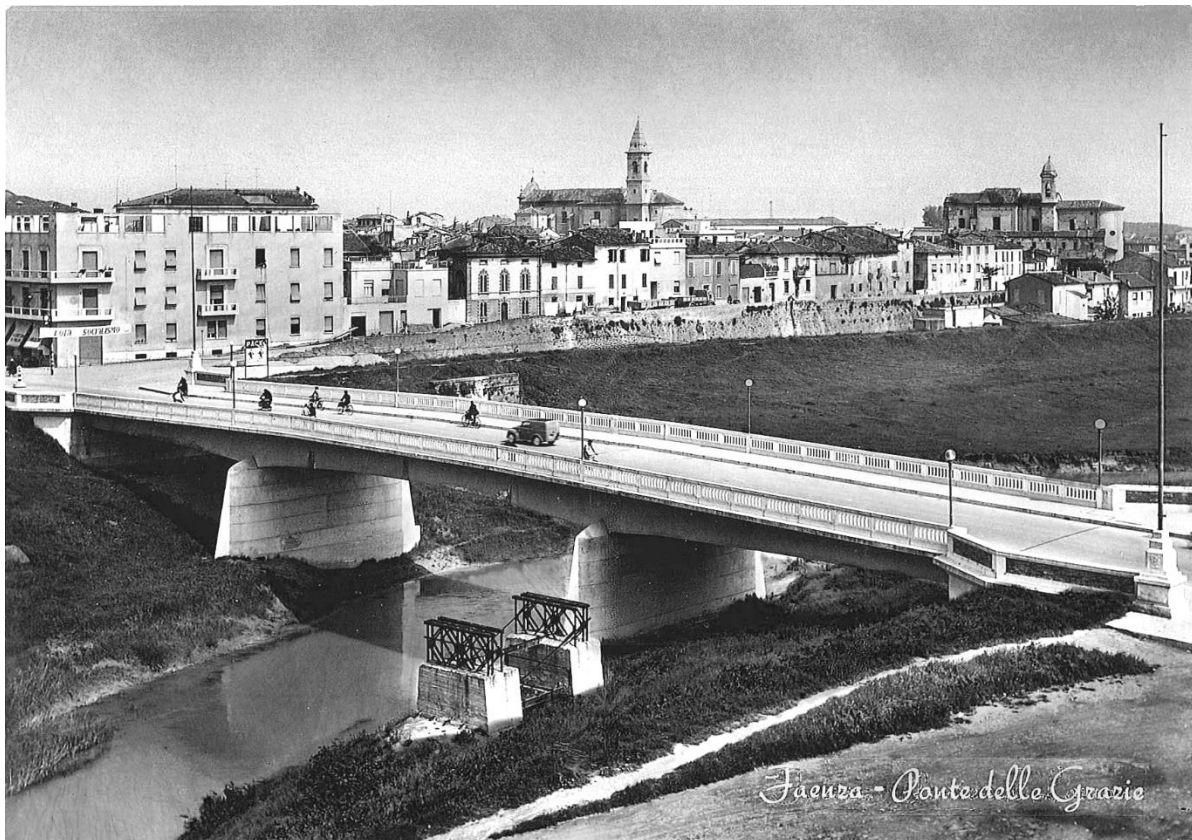
Figure 1. The “Ponte delle Grazie” bridge located on the Lamone River in an original postcard.
