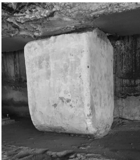
Figure 15. Reinforced concrete bearing after concrete reconstruction.
