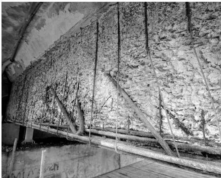
Figure 11. The main beams after the cleaning with hydro-scarification.
