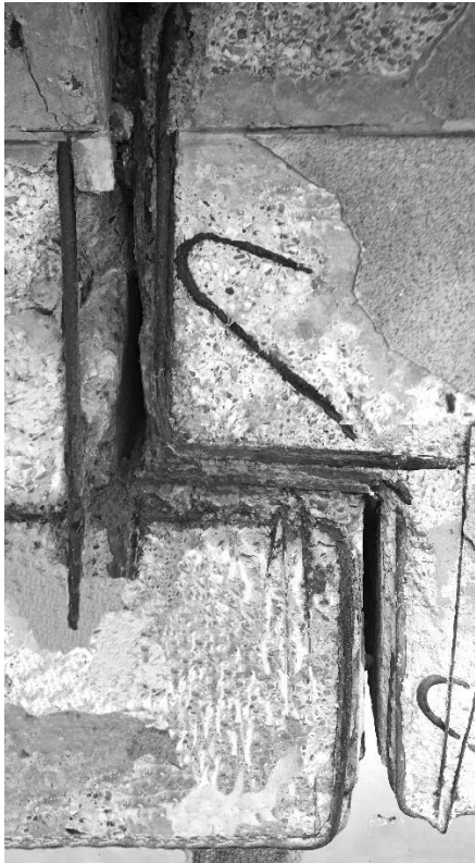
Figure 7. Gerber half joint at actual state
