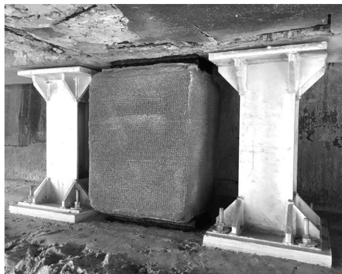
Figure 16. Concrete bearing after wrapping with FRP and the steel protections.
