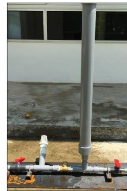
Figure 4. Adjustable waste valve installed at hydram
