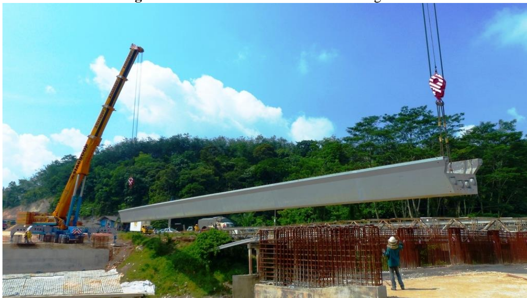
Figure 3. Typical view of UHPFRC precast/prestressed U-girder.
