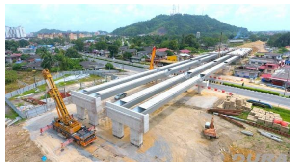
(h) All UHPFRC U-girders were launched
