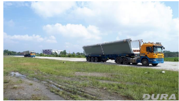
(b) Transporting U-girder segments using trailer
