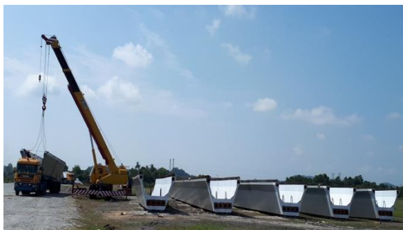
(c) Unloading and assembly of U-girders
