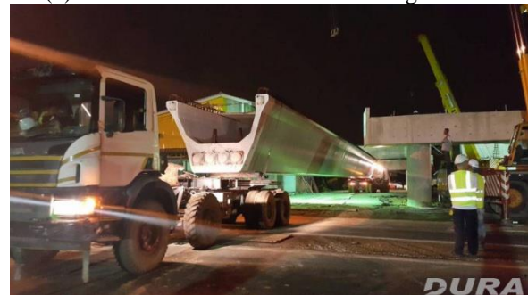
(f) Transporting U-girder for beam launching
