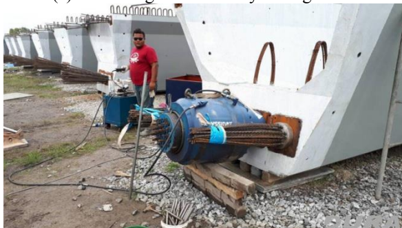
(e) Post-tensioning of tendons in progress
