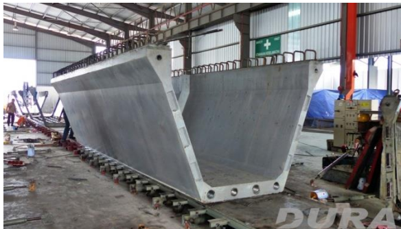
(a) Casting of 8m long internal U-segment
