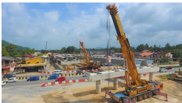
(g) 2 units 160 tonnes mobile cranes used
