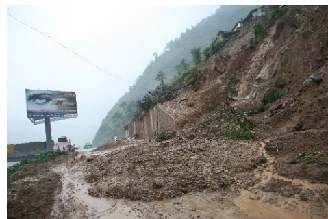
Fig. 2 Road destruction by debris flow
