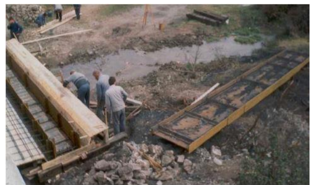
Figure 13. Cutting the existing structure and embedding it into a new one filled beams
