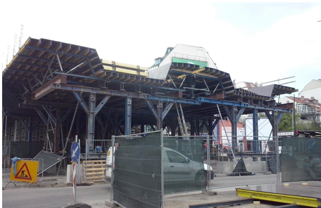
Figure 1. Densely placed scaffolding and limiting the traffic during the execution of a bridge of prestressed concrete at crossroad with heavy traffic in Sofia – 2014.
