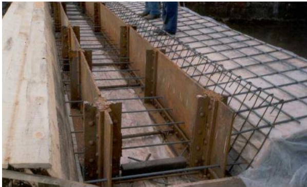
Figure 14. Beams and "soft" reinforcement of semi - structure
