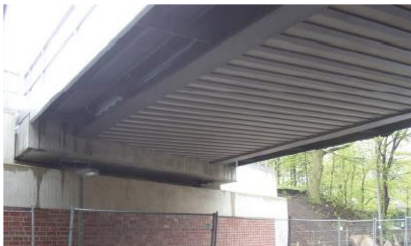
Figure 3. Railway bridge superstructure from imbedded steel profiles in transversal direction
