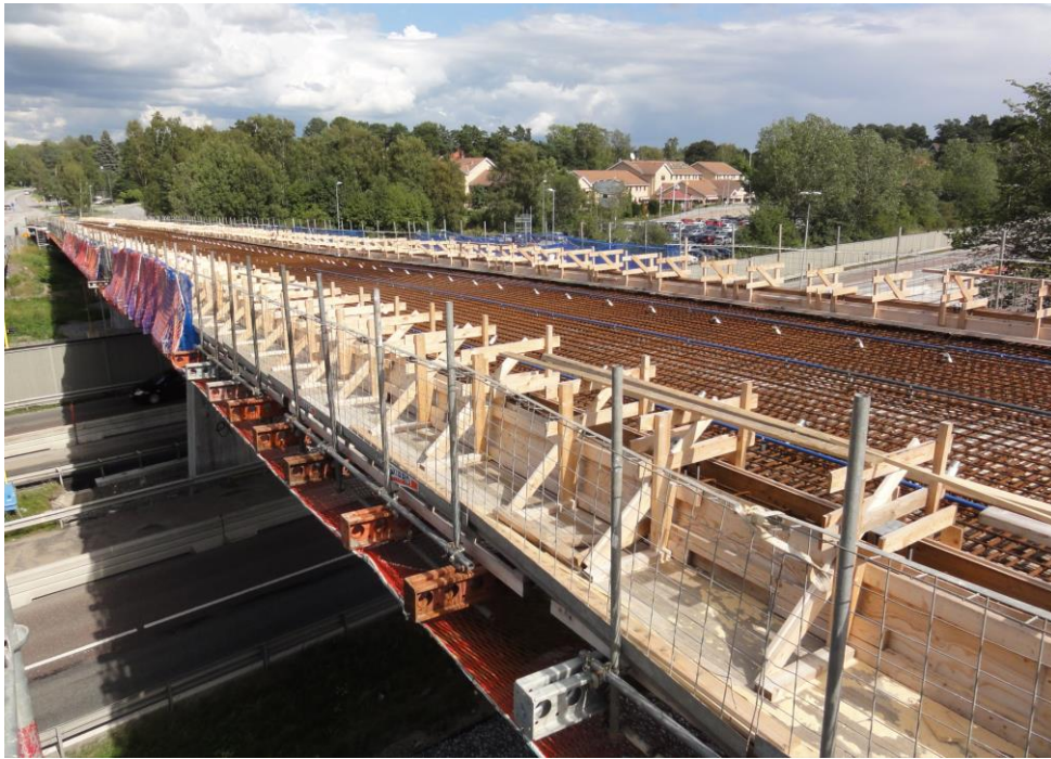
Figure 8. Unshored formwork of the concrete slab.
