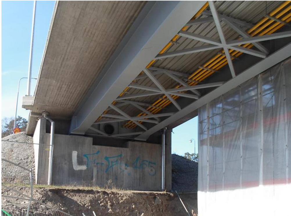
Figure 4. Diaphragm, intermediate stiffeners and diamond-bracing.
