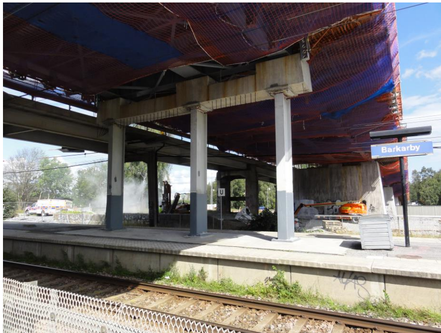
Figure 5. First stage of support 4 and unshored erection of deck.
