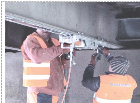
Figure 4. Passive anchorage mounted on the steel beam
