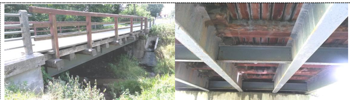
Figure 3. The steel bridge before strengthening.
