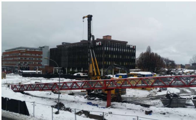
Figure 14. Work on pile-drilling in the southwestern quarter of the construction site.
