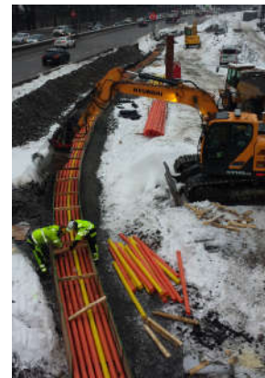
Figure 15. Work on relocating electrical cables in the ground.
