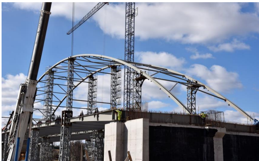
Figure 19. Construction of MS-15 bridge with 120 m span length in northern Poland, road S51 Olsztyn-Olsztynek, part Olsztyn East – Olsztyn South [8].
