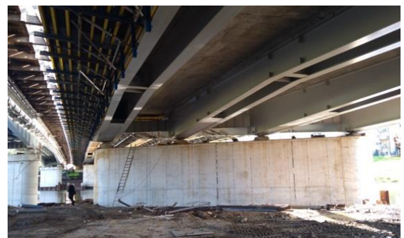
Figure 12. Bridge in Niemodlińska street in Opole: bottom view after construction of concrete slab.
