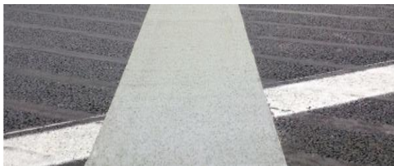
Figure 12. Poured polyurethane flexible plug joints such as the Polyflex joint offer many advantages over the traditional asphaltic type.
