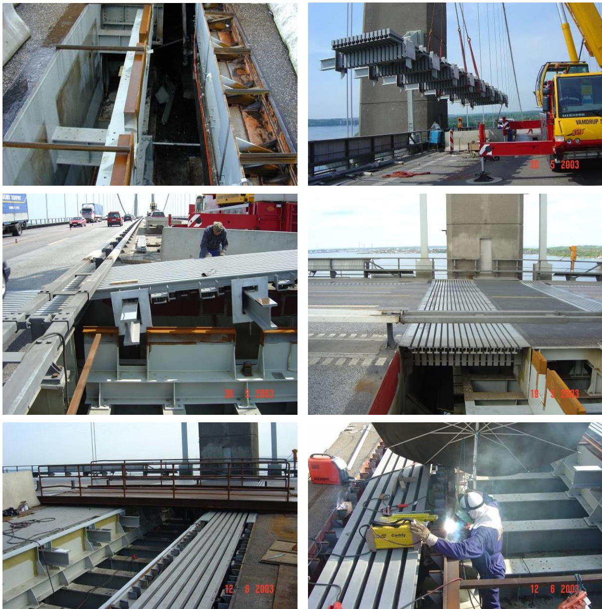
Figure 2. Installation of 7-gap and 14-gap Tensa-Modular expansion joints, side by side, during renovation of the Lillebaelt Bridge, Denmark (2002).
