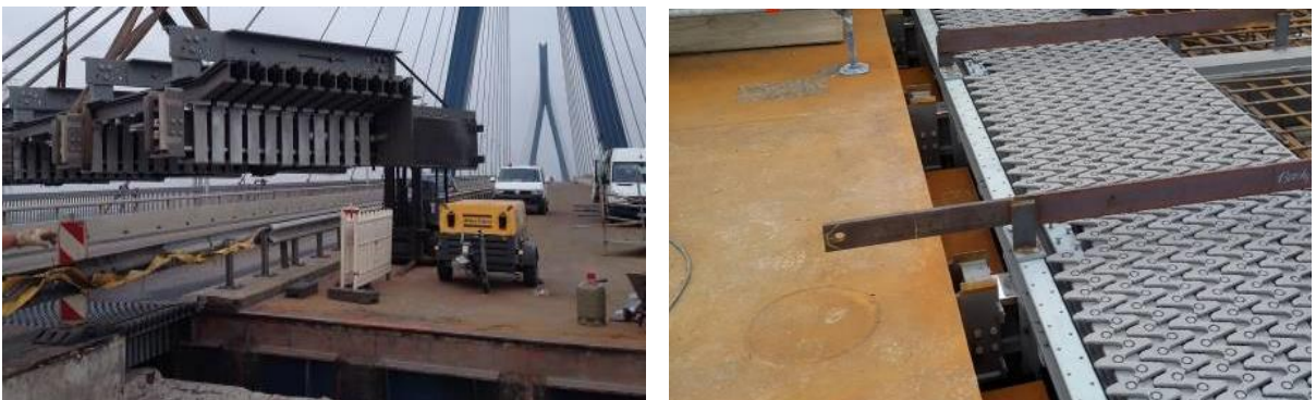
Figure 5. Installation of a 12-gap Tensa-Modular expansion joint with noise reducing “sinus plates” on its surface on the Köhlbrand Bridge, Hamburg, Germany (2016).
