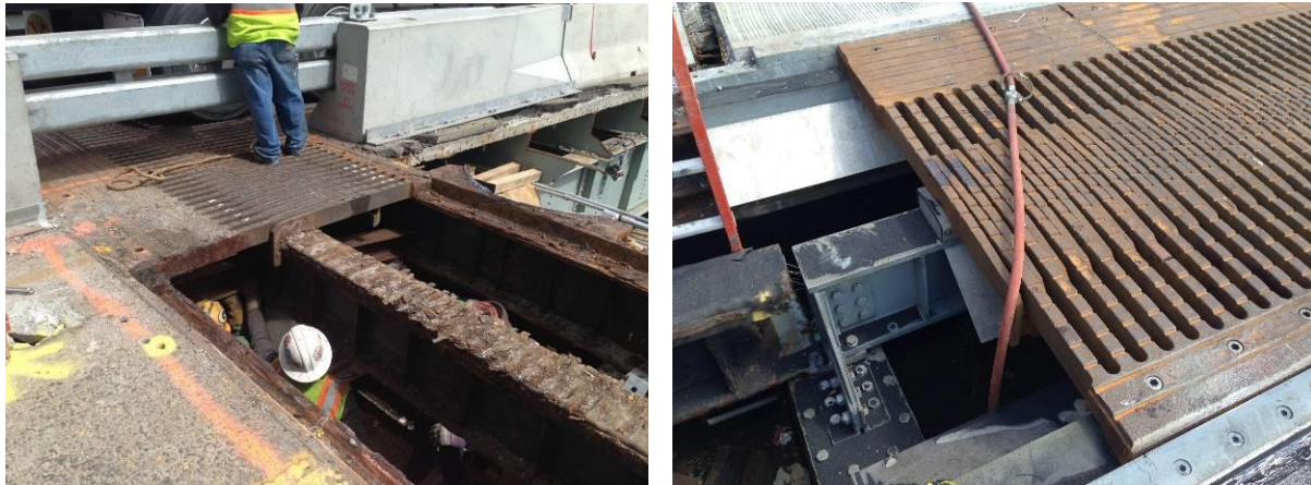
Figure 7. Replacement of Tensa-Finger sliding finger expansion joints with movement capacities of up to 2700 mm in the Verrazano Narrows Bridge, New York, USA (2017).
