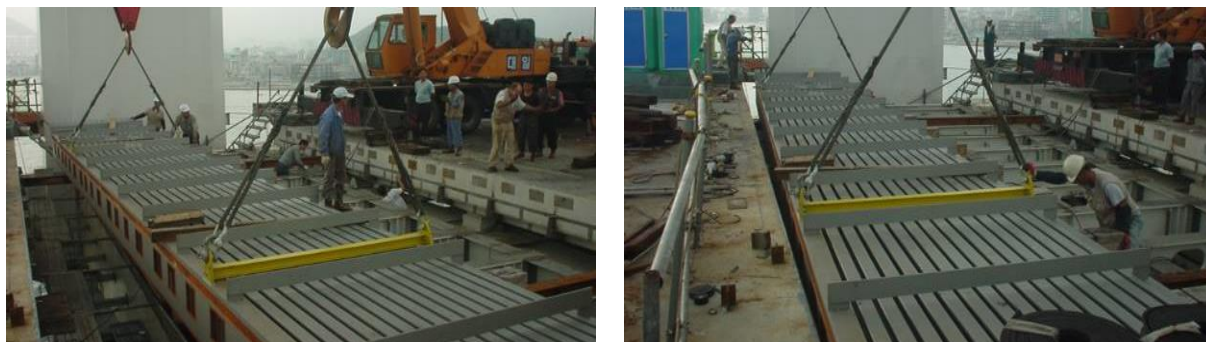
Figure 3. Installation of a 15-gap Tensa-Modular expansion joint during construction of the Guangan Bridge, Busan, South Korea (2002).
