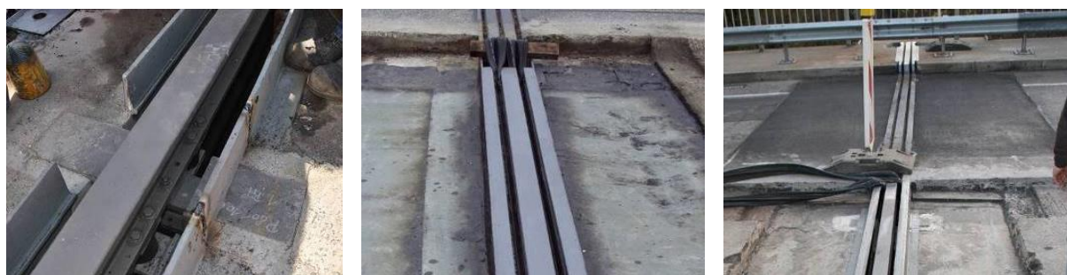
Figure 10. “Box-in-Box” method (cont.): Reinstatement of edgebeams where cut (with recesses for rubber seals); Insertion of rubber seals; Reinstatement of road surfacing – if needed, one lane at a time.
