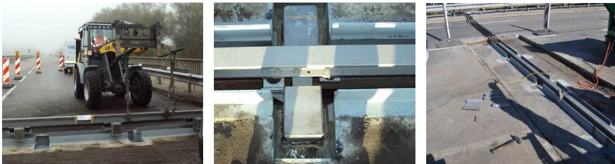
Figure 9. “Box-in-Box” method (cont.): Lifting in of new structure consisting of centerbeams and support bars; Welding of new box inside old box; Concreting of spaces between new and old boxes.
