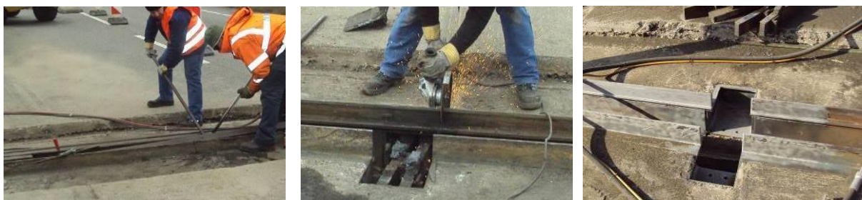
Figure 8. Renewal of a Tensa-Modular expansion joint by the “Box-in-Box” method: Removal of rubber seals and steel centerbeams; Cutting of edgebeams; and removal of transverse support bars.
