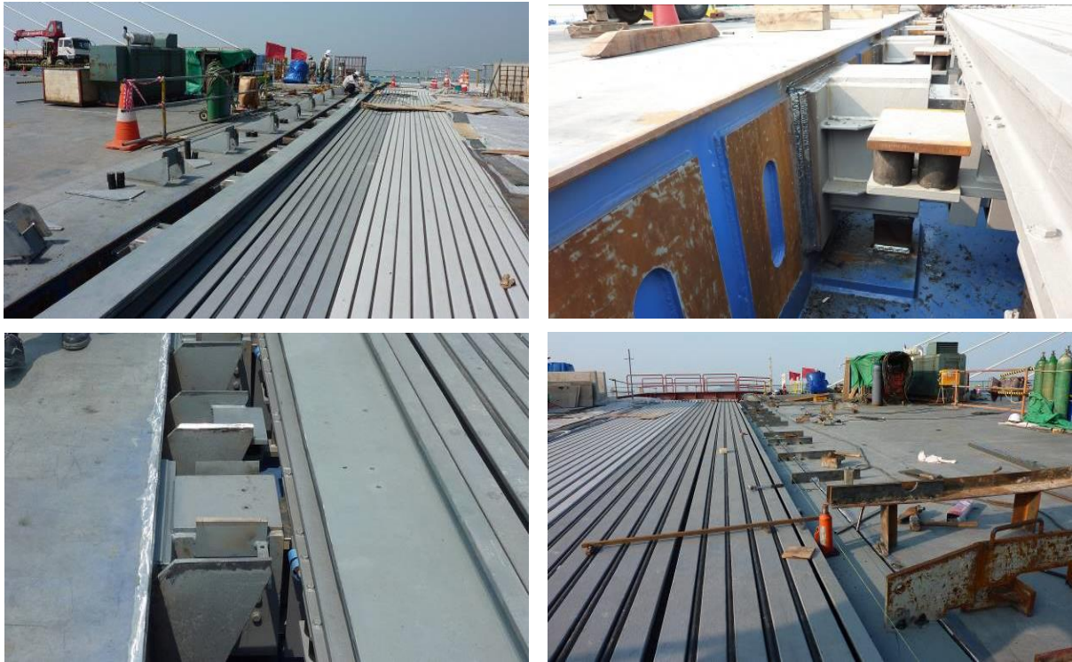
Figure 4. Installation of a 24-gap Tensa-Modular expansion joint during construction of the Incheon Grand Bridge, South Korea (2008).
