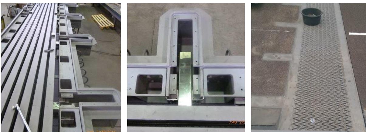
Figure 11. A Tensa-Modular expansion joint as specially designed for easy future renewal by means of the “Quick-Ex” method – maintaining the joint’s connections to the main structure.
