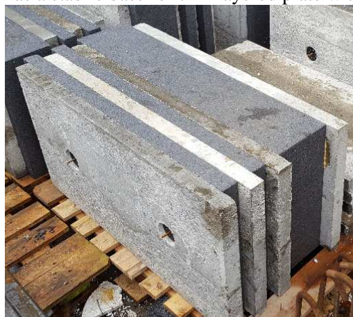
Figure 2. Ekoblok wall system elements.
