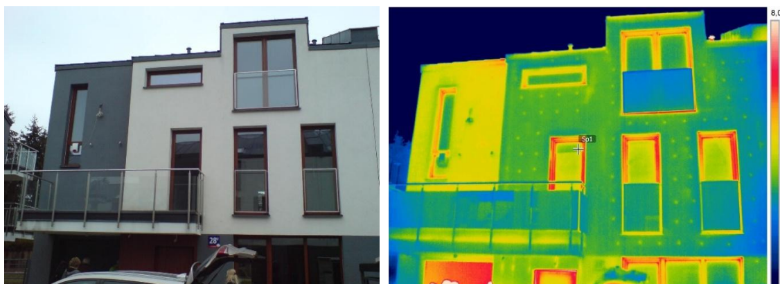
Figure 3. Thermogram and photo of the building in the NF40 standard - front elevation (S).
