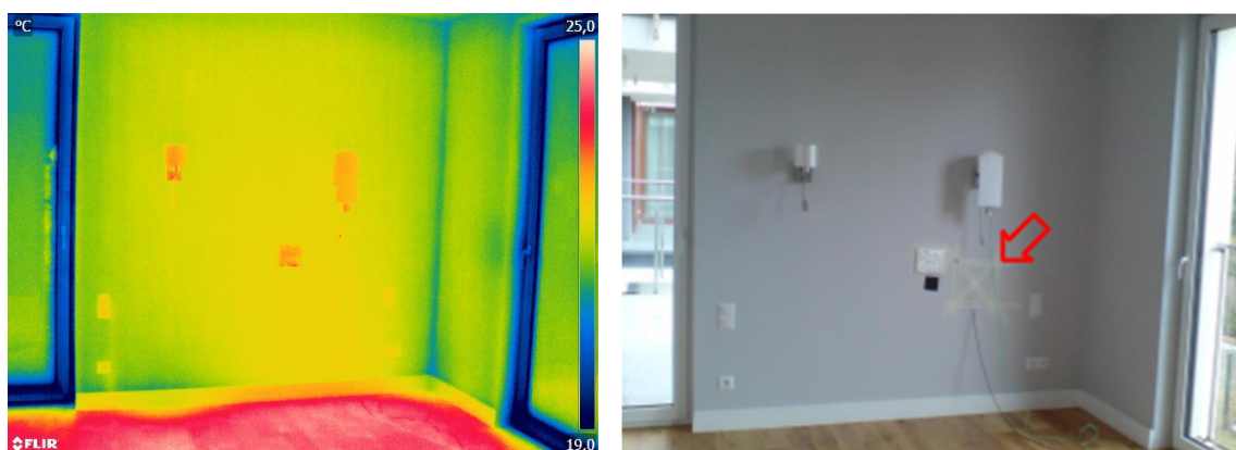
Figure 5. The location of the heat meter on the tested western wall of the NF40 building (1) - a thermogram and photo.
