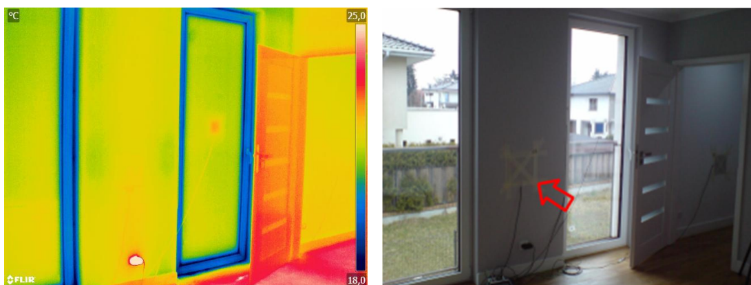
Figure 7. Heat meter on the tested northern wall of the LE (1) building (pier between window openings) - thermogram and photo.
