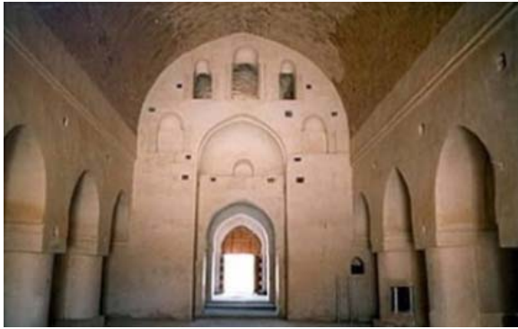
Figure 1. Pointed barrel vault and arches of the great hall of Al-Ukhaidhir Palace – Source: https://www.cemml.colostate.edu
