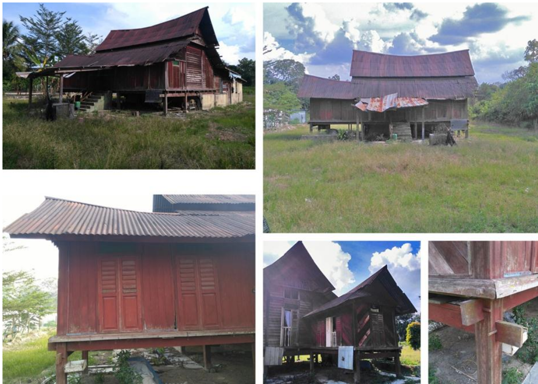
Figure 2: Views of Raja Kamarudin's house and its joint of pillar, beam and floor joist (lower right)
