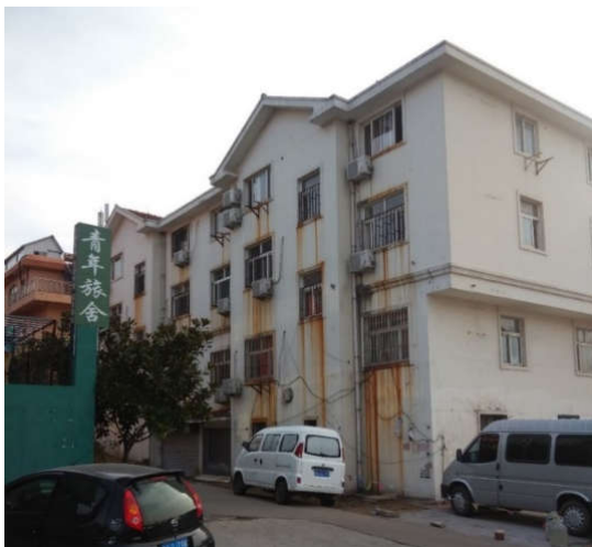
Figure 13. Ferruginous leaks. Expression of material deficiency.
