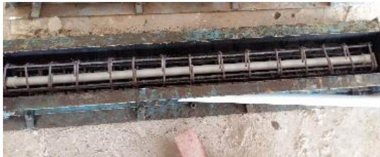
Fig:2: Reinforcement cage of the beam
