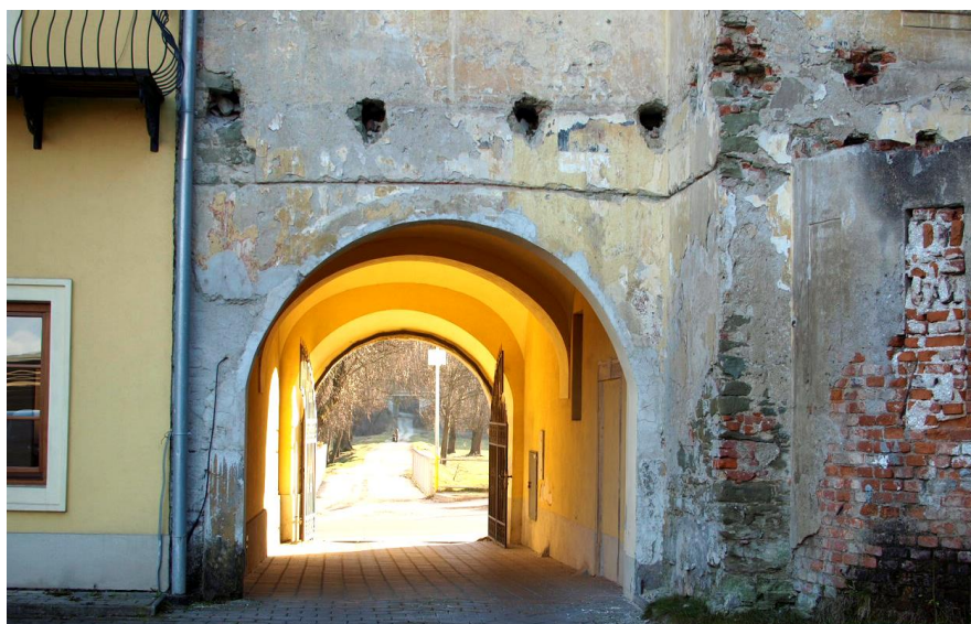
Figure 2. Damaged part of east side of façade, damp, salinity and biocorrosion ( owner photo ).
