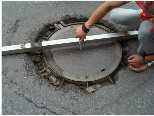
Figure 1. Inspection well subsidence
