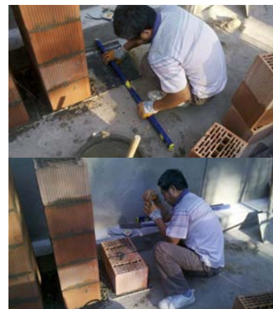
(b) Construction process
