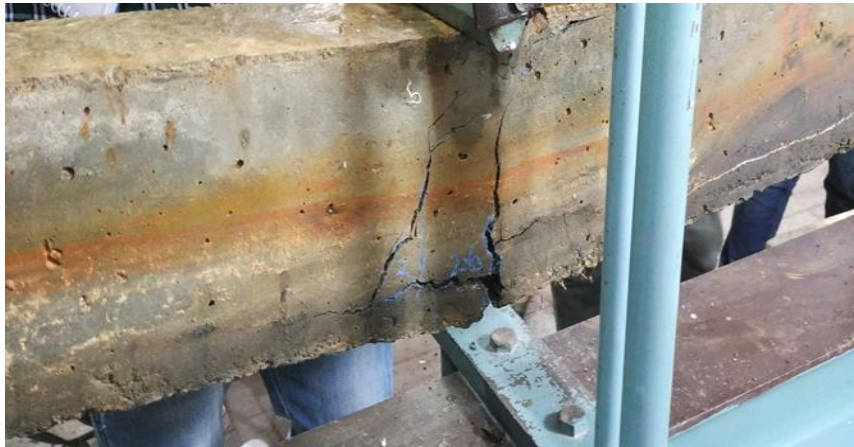
Fig 4. Bond failure due to corrosion
