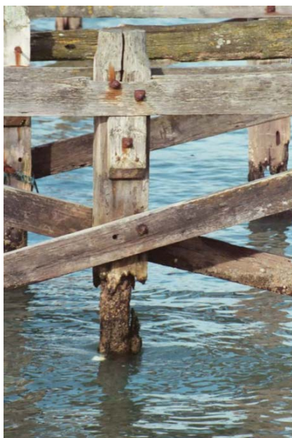
Figure 1. Degraded wooden pile [6]. Figure 2. Proposed solution – mixed wooden-concrete piles.
