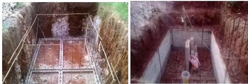
Figure 8 Installation of sloof beam reinforcement floors and wall of pond.
