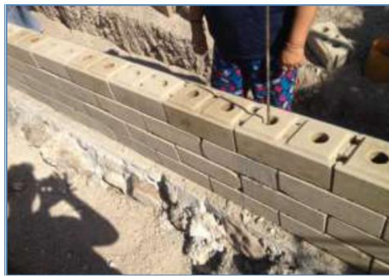
Figure 3 Arrange the walls of the building and prepare the iron for the column
