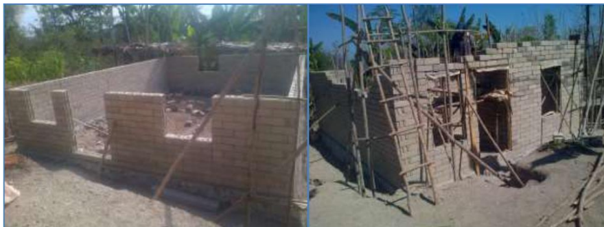
Figure 4 Installation of lock-brick wall, door and window holes
