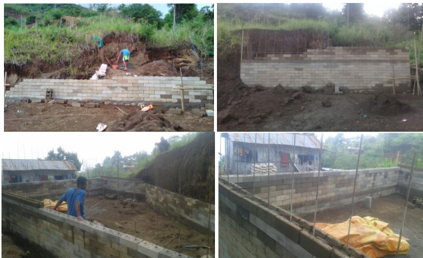
Figure 9 Installation of up-ground pond wall
