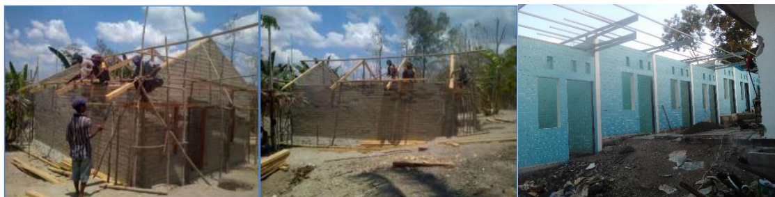
Figure 6 Implementation of roof installation work
