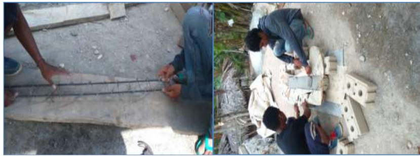
Figure 5 Construct concrete reinforcement for latei-beam
