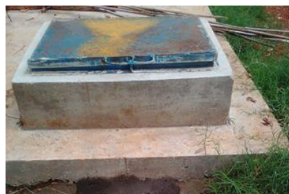
Figure 10 Concrete slab for the top of the pond
