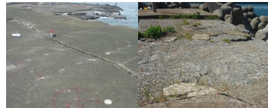
Figure 2. Deterioration of fishing port facilities.
