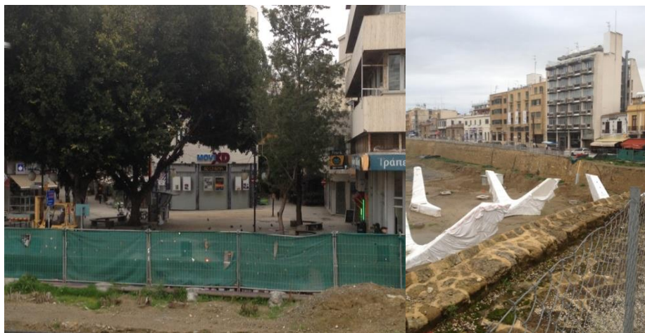
Figure 14, 15. Ledras from different angles and street levels.
