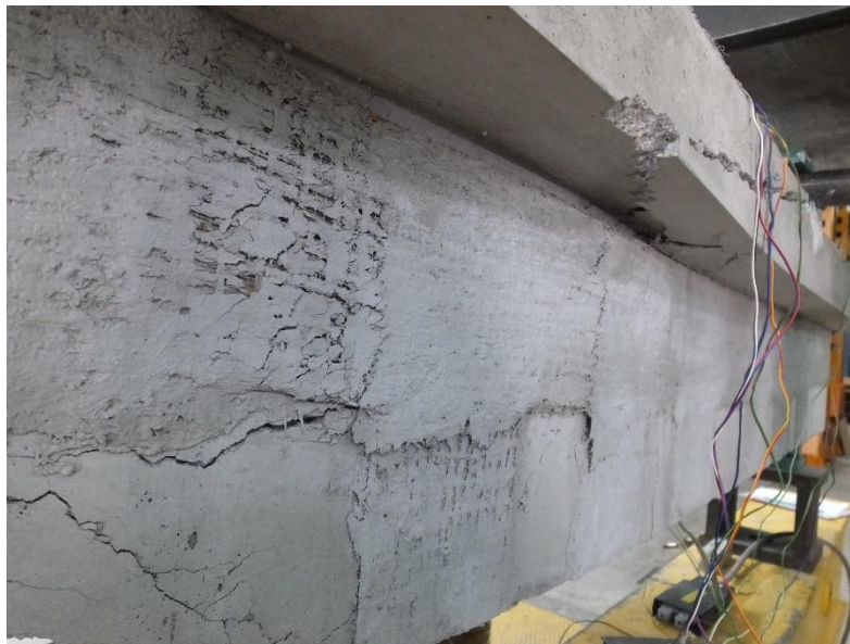
Figure 7. B_W1 failure. Vertical cracks at the edge of the vertical strips and slippage of the fibers at the ends of the longitudinal PBO strip, beyond the supports
