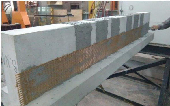
Figure 3. PBO strip application along the beam under the slab
