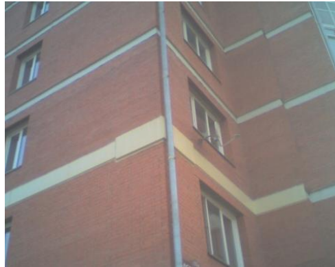
Figure 5. The supplementary thermal insulation layer
